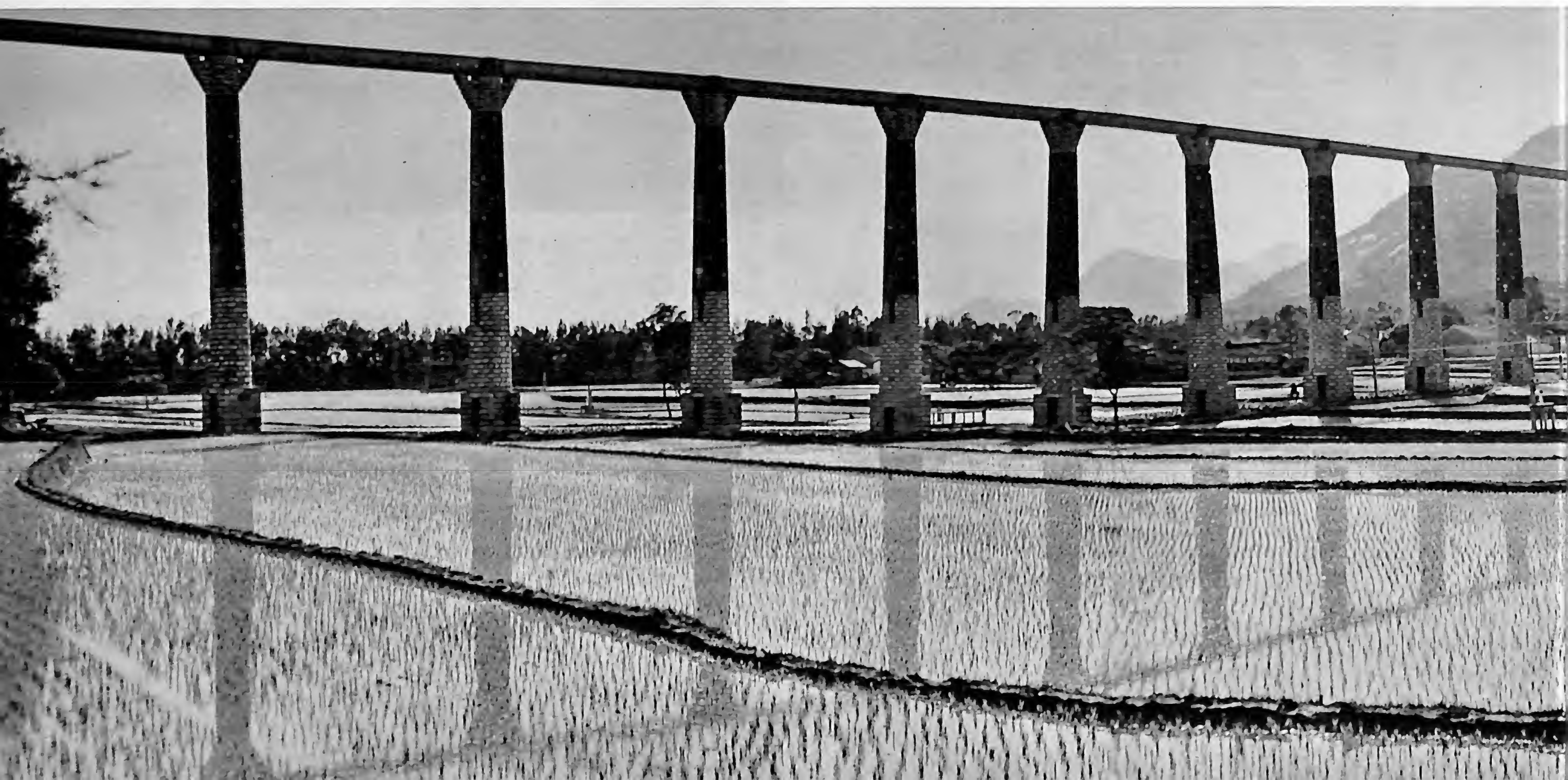
The 510-metre-long Hsiangtung Aqueduct is 18 metres high. It is one of the water conservancy structures built by the Chiaomei commune.
